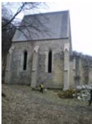
The new roof
