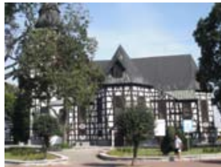
St Andrzej Bobola – This is actually in Milicz where we stayed and is a photo of a 300 year old church originally built as a protestant church in a predominately catholic country. Consequently they were only allowed to build it providing it could be pulled down. It, therefore, lacks nails!
